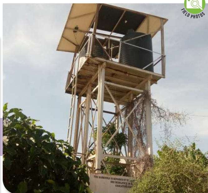
Revamped School borehole and water storage tanks, Nigeria
