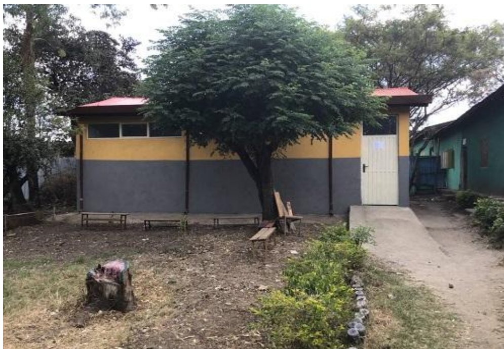
Picture 8: SNE Training and Assessment Center built by the project in Bishoftu city at Tokuma School
